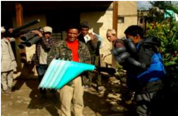
Carrying toilet construction materials
